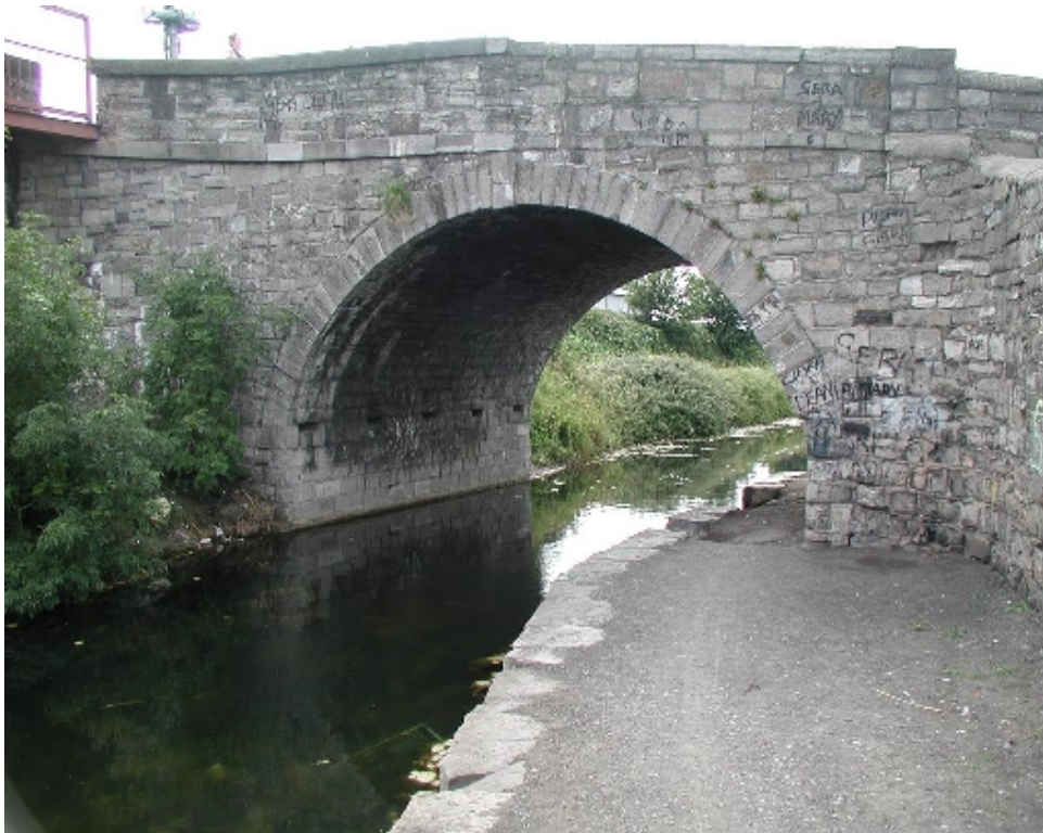
Brougham Bridge, Dublin
